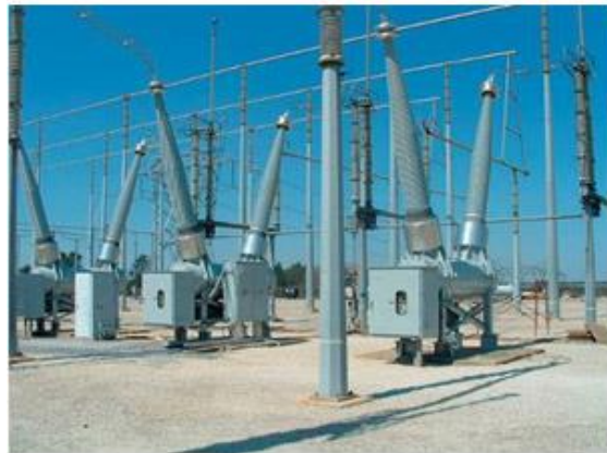
500 kV gas breaker
