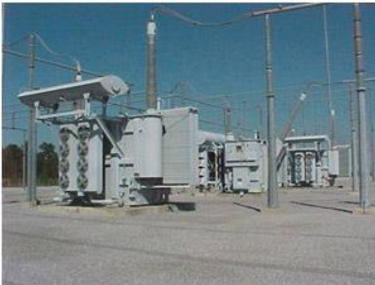
500 kV to 230 kV single-phase transformer
