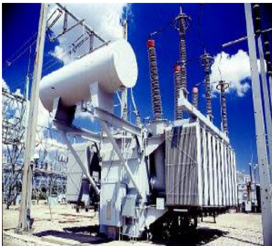
Step-Down Transformer © 2011, OSHA
