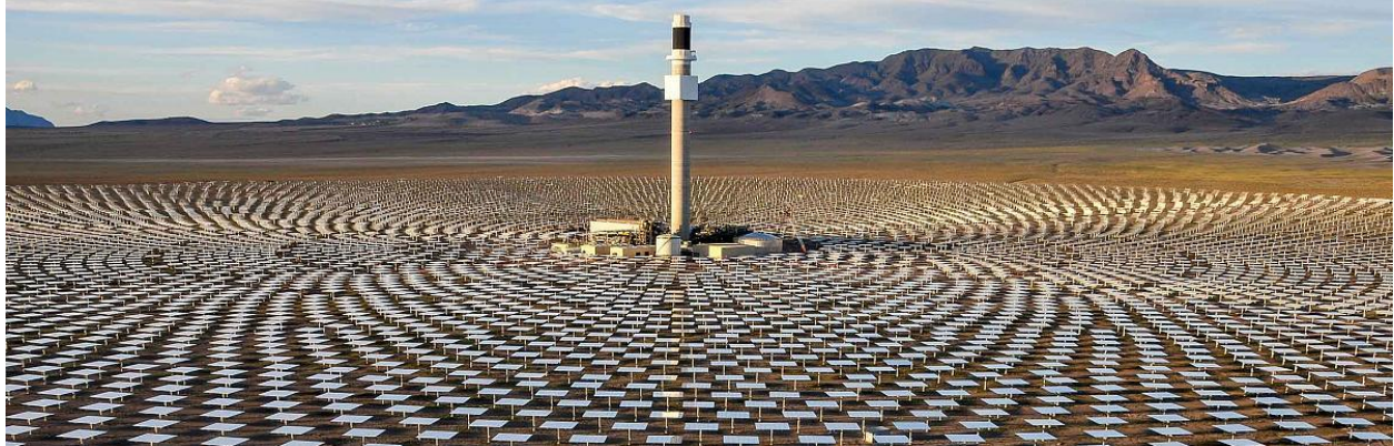
Figure 3C.6 Power tower system
