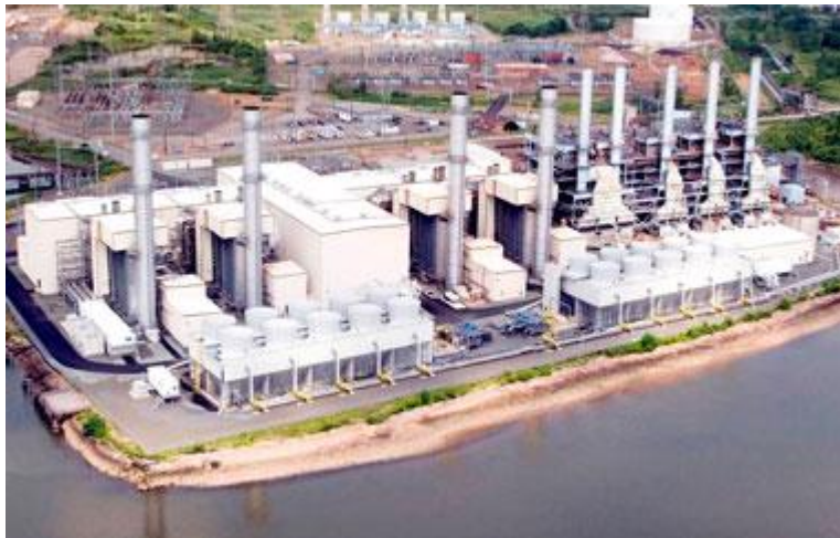
Linden Generating Station
